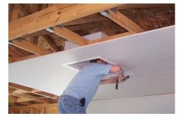
"Tack" nail frame in place with drywall nails
