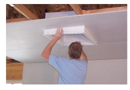
Remove Skuttle door from frame and slide frame into rough opening Note: It is easier to place door in attic prior to installing frame
