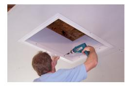
Install 2 1/2" drywall screws through predrilled holes. Note: Do not over tighten & shim as needed
