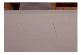
Texture the door and frame the same as you would the ceiling. Make sure to remove any dust from door prior.
