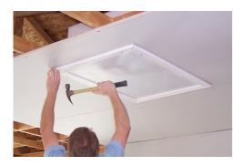
Option: if installing in existing homes you can install optional molding over nailing fin
