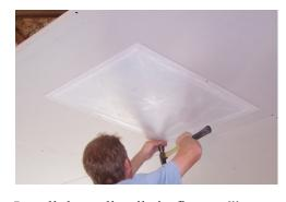
Install drywall nails in flange 6" apart
