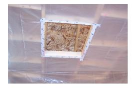
Install vapor barrier and seal to the framing
