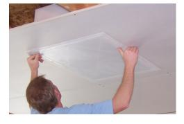
Check for even reveals around door and that when the screws were installed the side walls didn't bow
